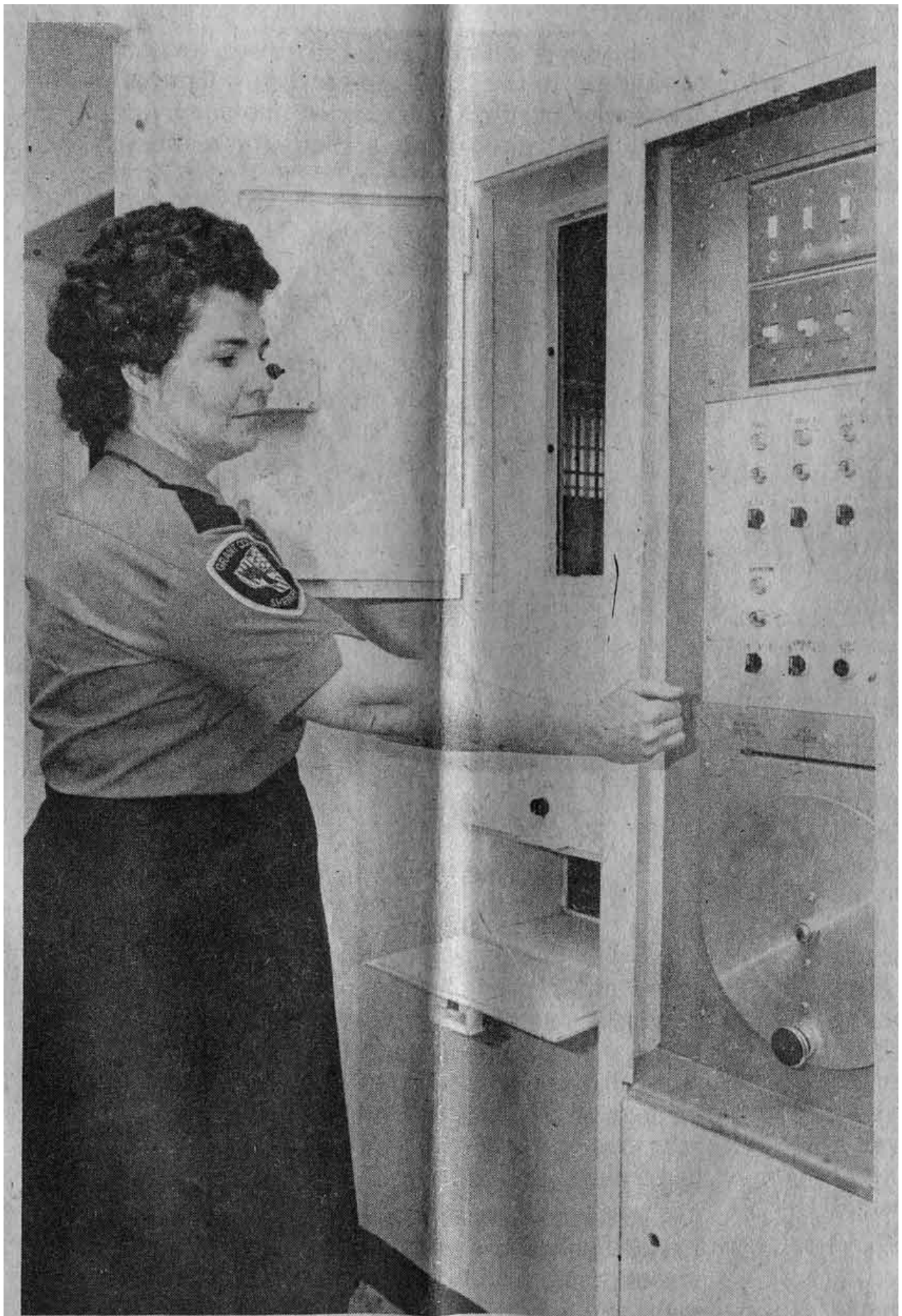
OFFICER LaVON BARTELS operates one of cell block control panels.
